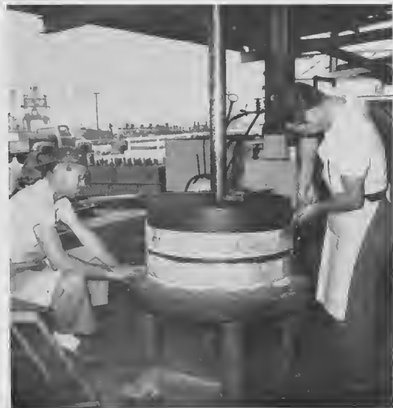
VARIETY OF Machine Shop tasks includes babbiting as performed here by H. Kelly, left, and S. de Cuba. Babbiting serves as a wiper ring for Edeleanu Plant compressor piston. E VARIEDAD di trabaonan den Machine Shop ta inclui "babbiting" cu cual H. Kelly, robéz, y S. de Cuba ta trahando aki. Babbiting ta sirbi como un wiper ring pa piston di compresor pa Edeleanu Plant.
